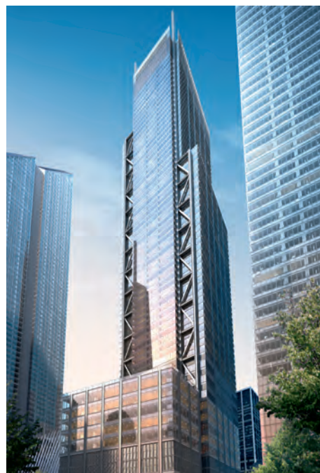
Equipped with building controls by Automated Logic, 3 World Trade Center will be one of New York City's greenest skyscrapers.
